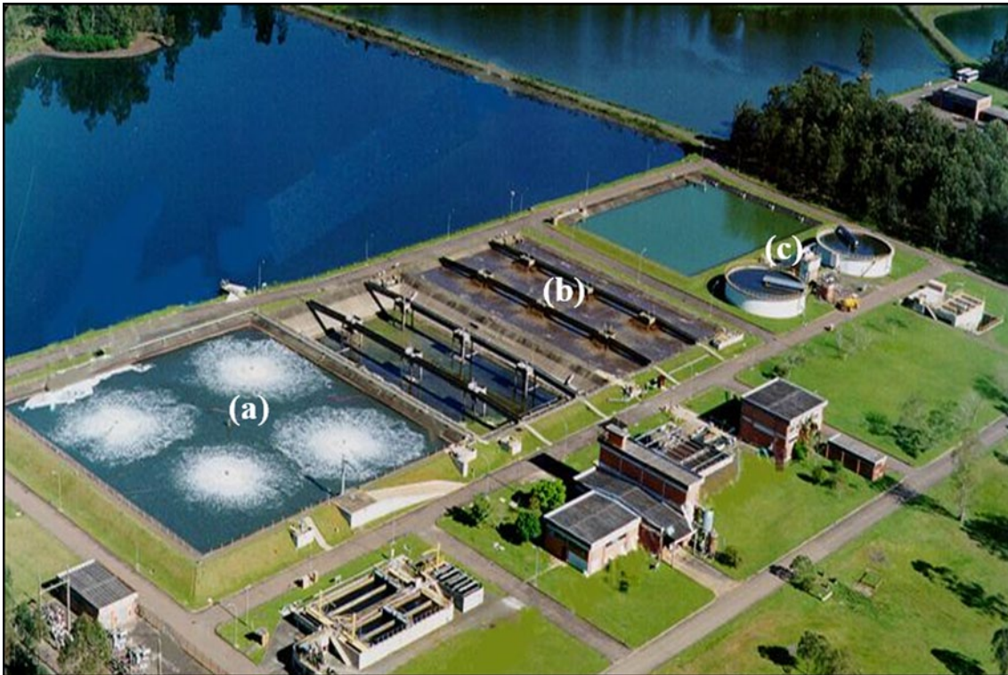
Fig. 1 Aerial view of the WWTP housing the equalization tank (a), the aeration tank (b), and the settling tanks (c)
